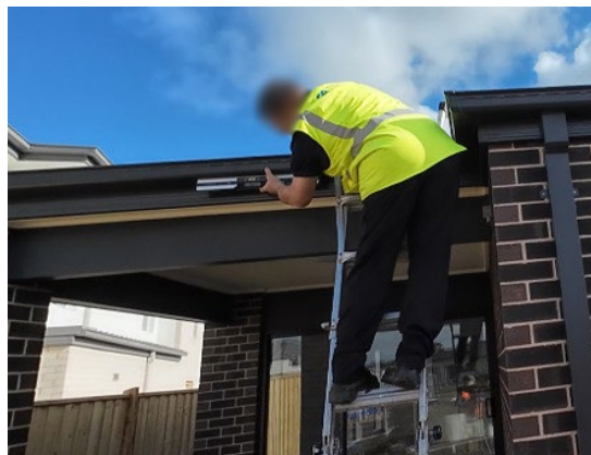
Figure 12: Inspector performing gutter gradient measurement in case study 2
