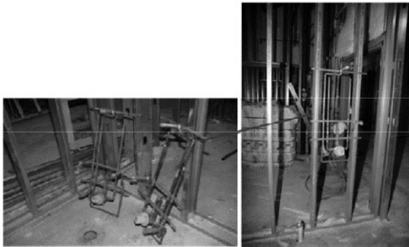
Figure 46. Pre-assembled piping Source: Kuprenas & Mock, 2009.
