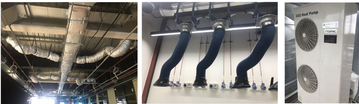
Figure 17. Internal insulated rigid and flexible ductworks
