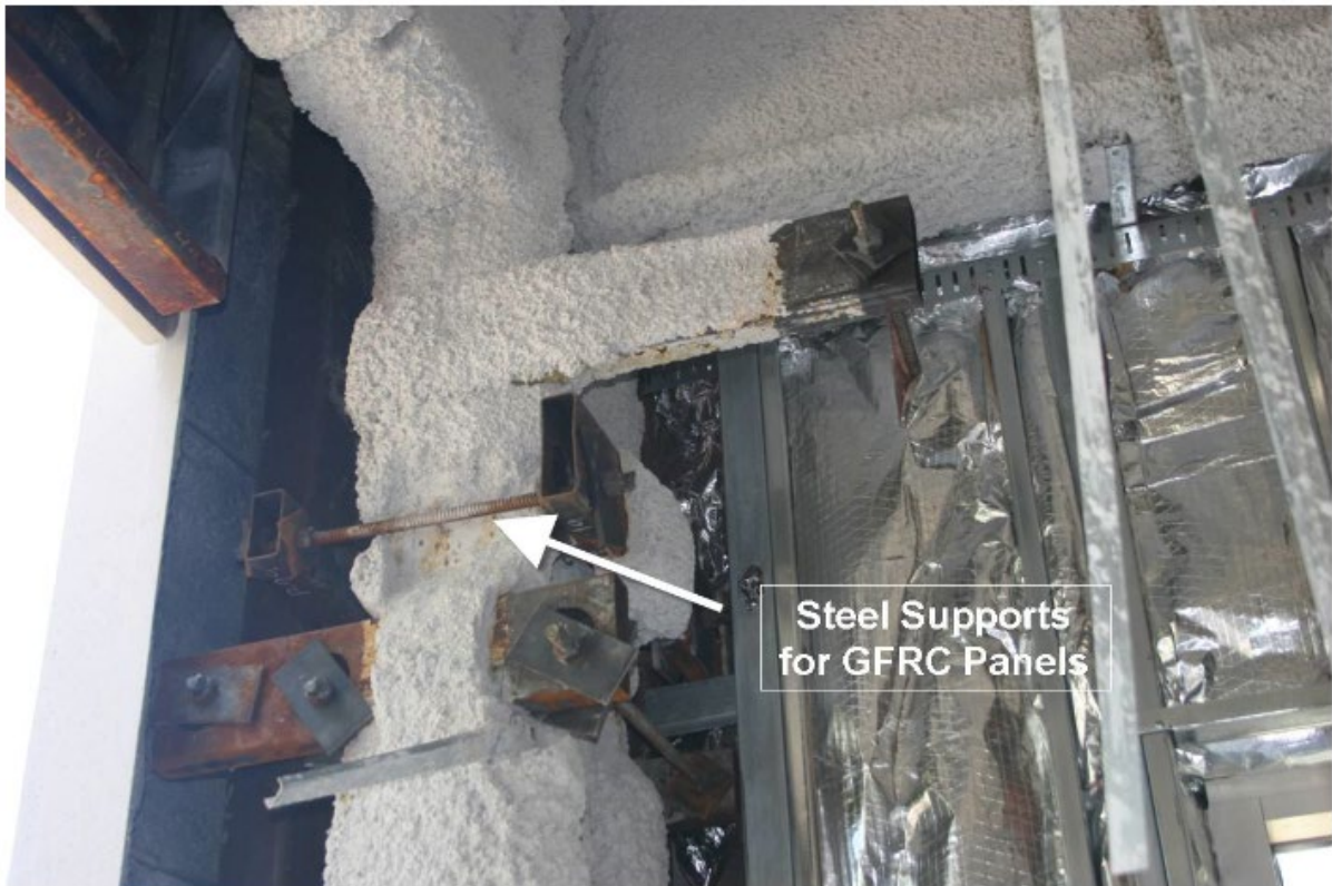
Figure 61. Conflict between the rainwater leaders and supports for the exterior glass fibre reinforced concrete panels Source: Khanzode et al, 2008.
