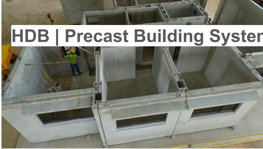
Fitting out of PPVC components off-site
