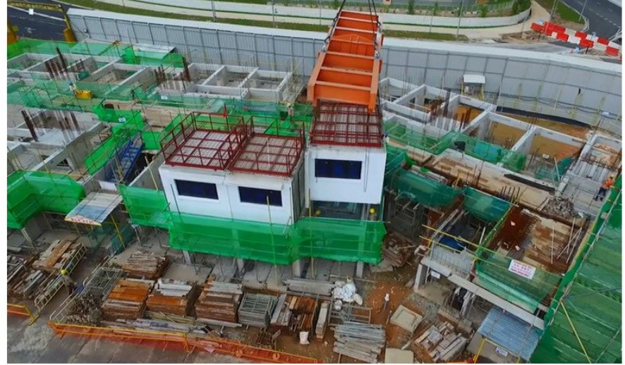
Hoisting of PPVC components
