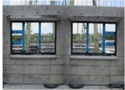
Fitting out of PPVC components off-site
