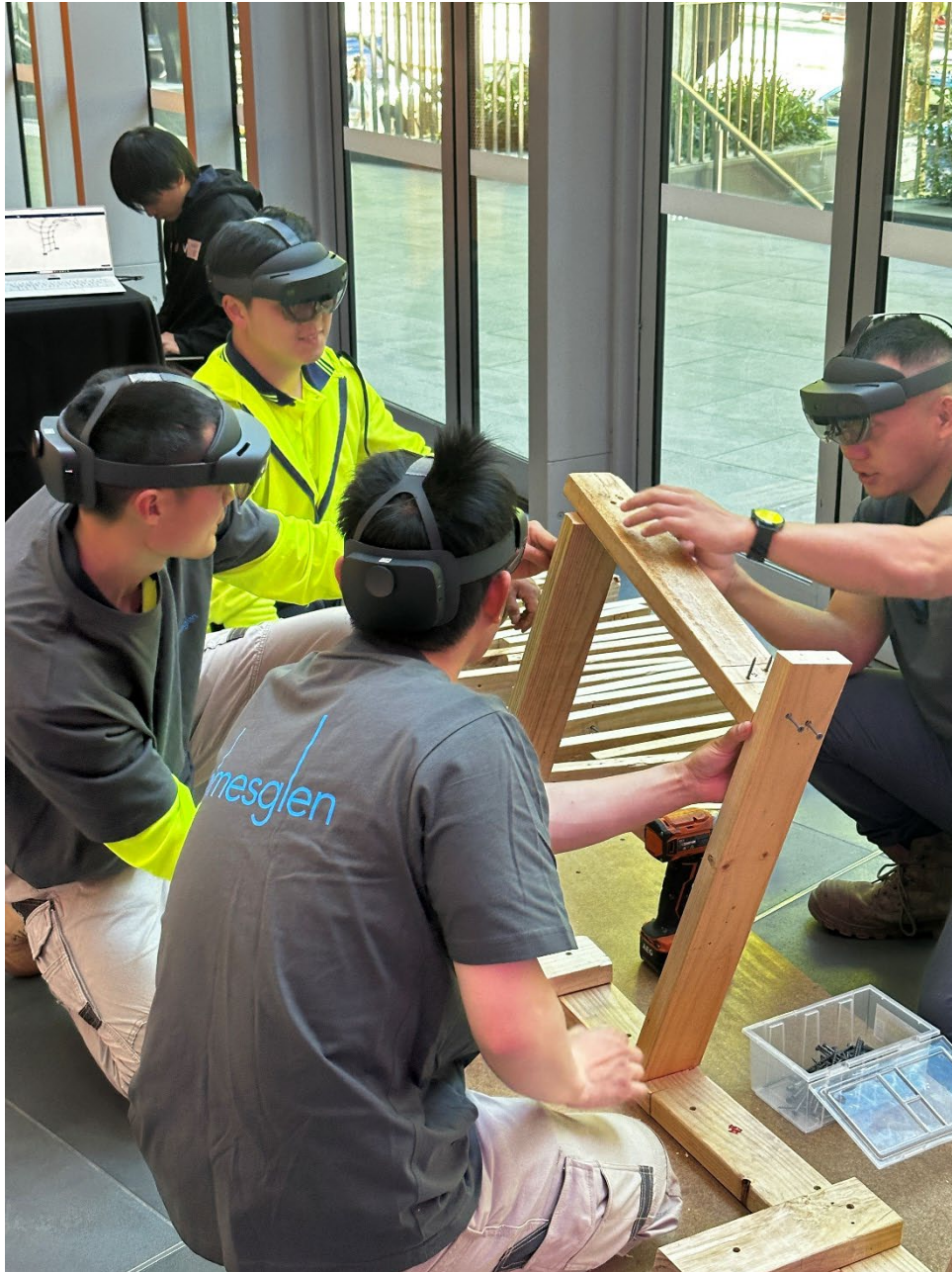
Figure 3. Carpentry students working on structure
