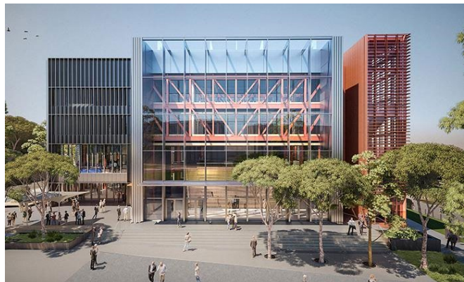
Figure 1. Design and Technology Building Monash University.
