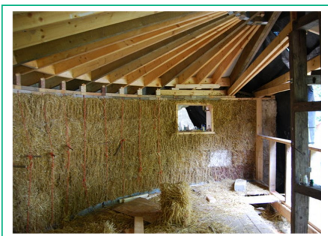
Figure 28. Straw bale house Source: Hayley Green (2009)
