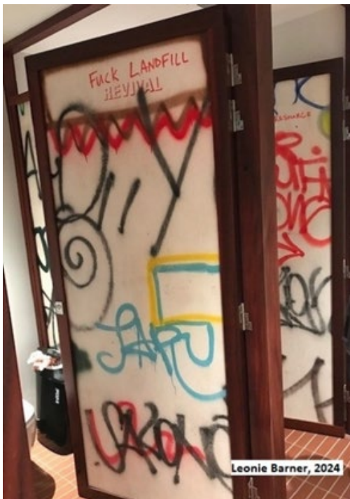
Doors of toilet stalls made from on-site salvaged hardwood and construction hoarding.
