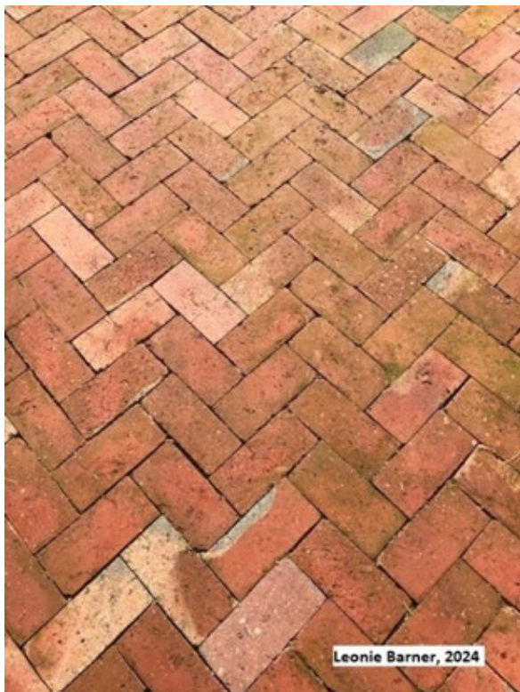
Courtyard pavement made from salvaged bricks.
