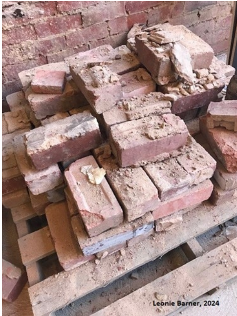
Examples of reuse: Bricks that had to be removed during the renovation were given a new life as pavement bricks for the courtyard.
