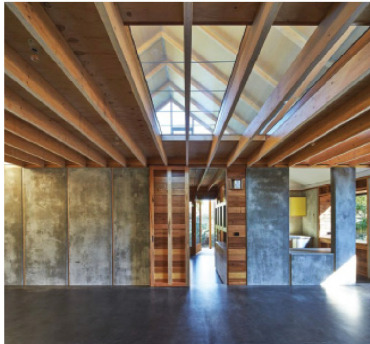
100% Fibre-based The base componentised wall system provides a high level of performance in fire, acoustic and thermal aspects.
