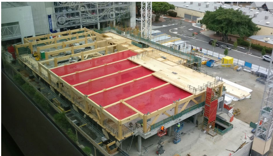
Figure 2: Construction process of level 2
