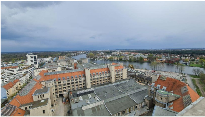
Figure 24. The Behrens-Ufer heritage factory buildings
