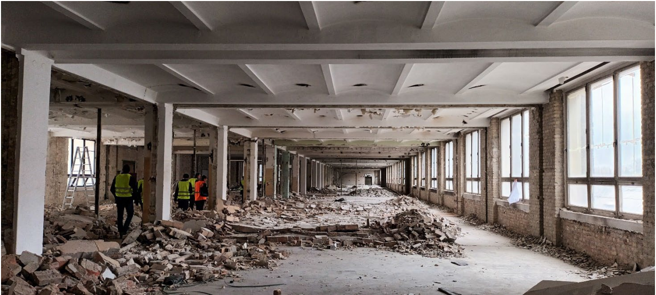
Figure 26. Heritage factory visit during construction works
