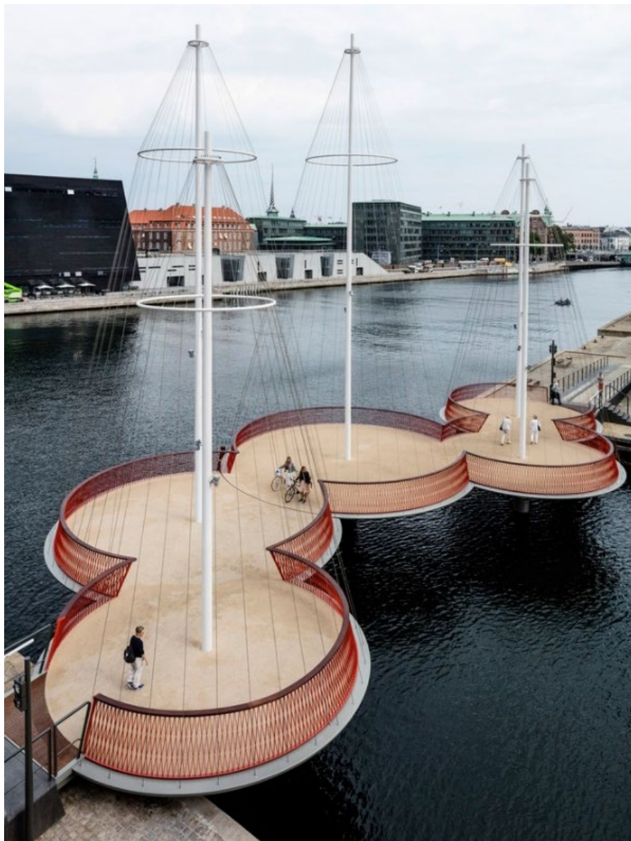
Figure 35. Cirkelbroen (The Circle Bridge)
