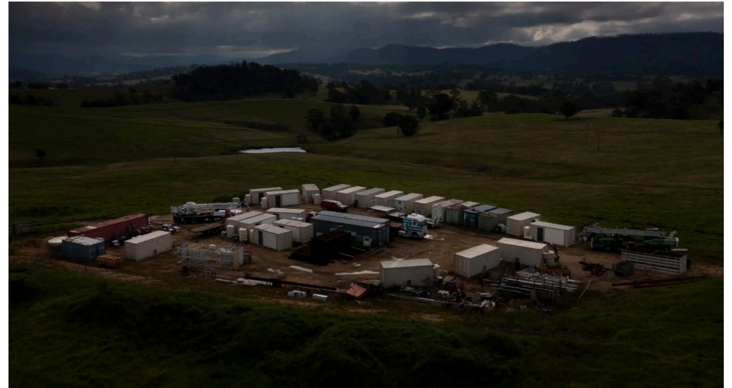
Figure 3: Temporary Accommodation pods ready to be deployed outside Cobargo. Image credit: New York Times
