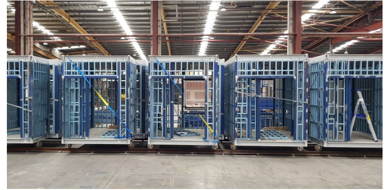
Image credit: Steel framed volumetric module assembly
