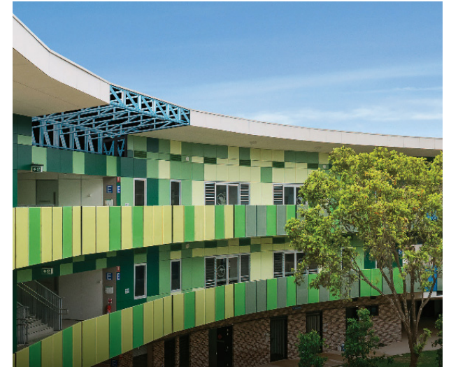
Image credit: Smalls Road Public School, Ryde, NSW. © School Infrastructure NSW and Austruss. Frame made from TRUECORE® steel.
